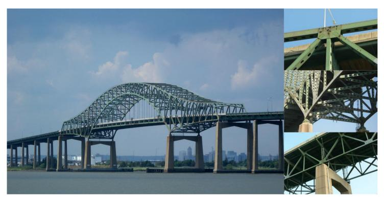
built in 1956 with 2003m total length, 207m maximum central span and 8 approaching spans from each side
